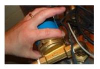
Now the pump is to be cleaned. Open the pump. It should be possible to open the pump casing by hand. If this is not the case, please loosen the union nut with a small squared timber and hammer.
