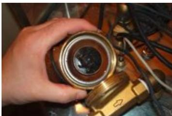
The rotor ball is now visible inside the pump. **Caution:** Rotor ball can fall out! Damage to the rotor blades will lead to subsequent failure of the pump!
