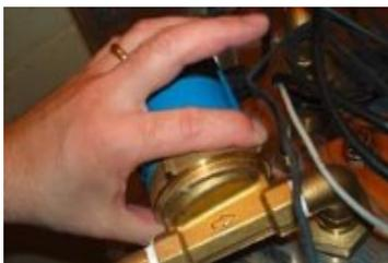
Now the pump is to be cleaned. Open the pump. It should be possible to open the pump casing by hand. If this is not the case, please loosen the union nut with a small squared timber and hammer.
